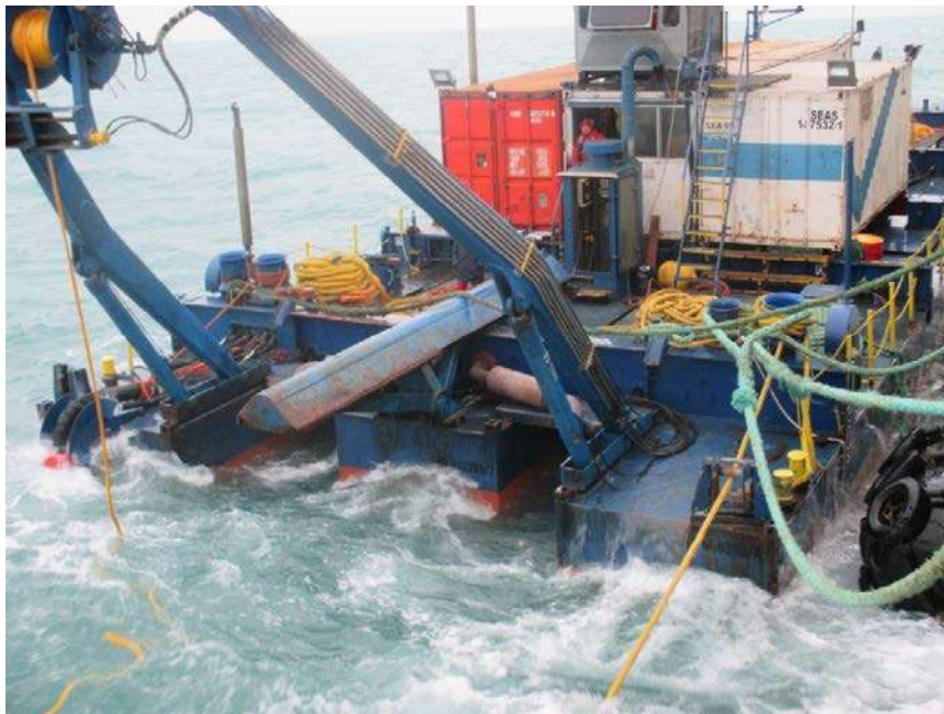
The Trimaran ROSSANA during the 2013 trenching activities
